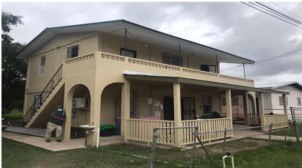
Renovation of Ladyville Health Center “Delivering on #Plan Belize”
