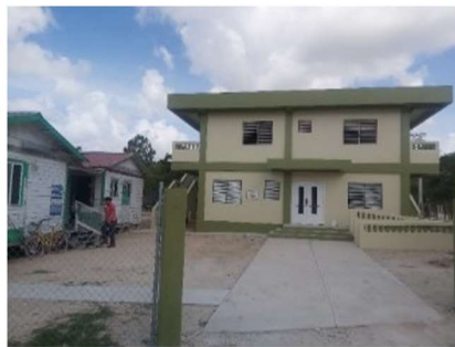
Image showing Belmopan, Caye Caulker and Crooked Tree Health Facilities- newly built
